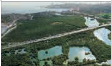
Existing : Mangroves and Bridge Blocking Water Flow
