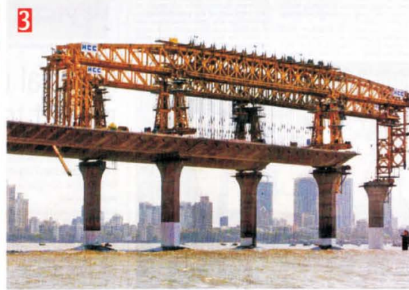
■ (Clockwise from Top) 1) A bird's eye view of the under-construction Bandra Worli Sea Link 2) The under-construction Bandra Worli Sea Link 3) A truss weighing 1250 MT places concrete spans on the sea link 4) Workers strike a pose in front of their work of labour 5) Construction workers prepare concrete sections
