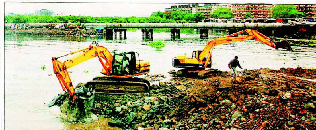
Desilting and widening of part of the Mithi was completed in the first phase. Work on Phase II has now been extended by three years. Source: Author
