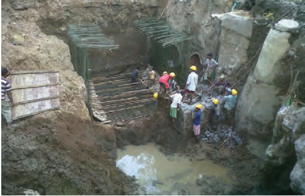
A part of the construction of box drain for BRIMSTOWAD
