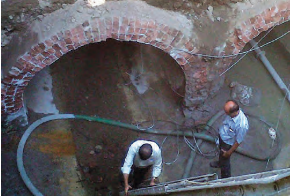
A part of the rehabilitation of arch drain for BRIMSTOWAD
